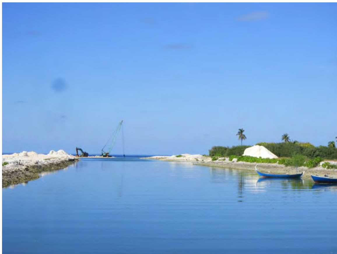
Figure 4.5: Project side during construction while attempts were made to dislodge the hard substrate using a 6 ton drop hammer
