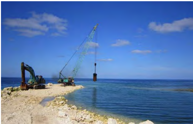
Figure 7.1: Drop hammer being used at the proposed site
