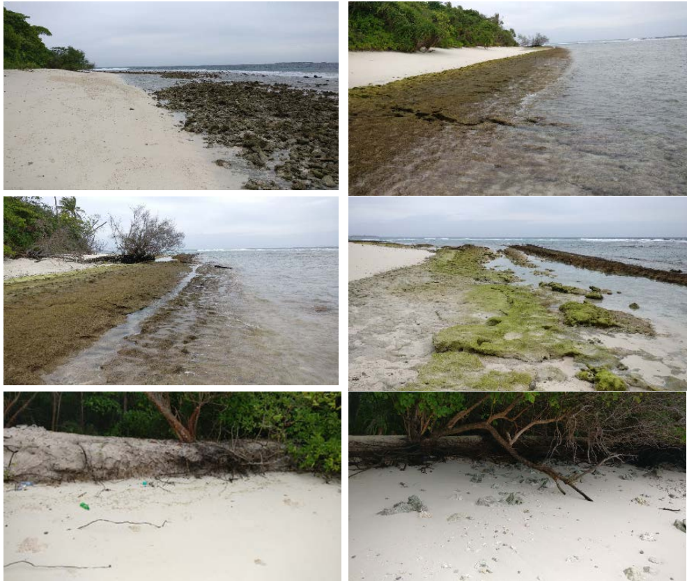
Figure 22: Severe erosion beach rock covering larger part of the western side of the island
