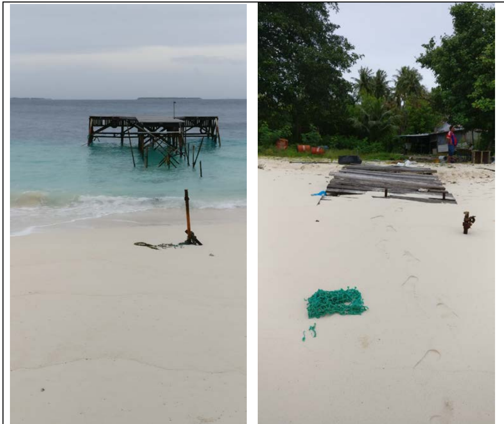
Figure 5: Condition of the existing jetty, looking seawards (left) and land wards (right)
