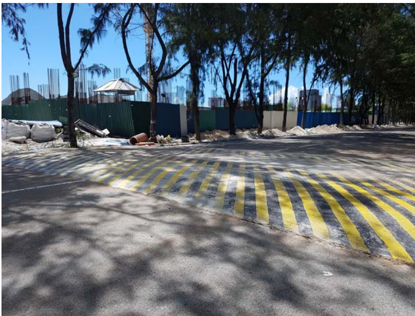
Figure 8 Speed breaker as protection for dewatering pipes
