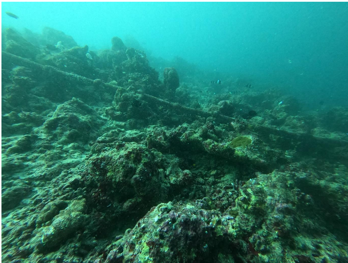
Figure 3. Submarine fibre optic cable at initial approved pipeline route (crossing the proposed pipeline route around 6m depth)
