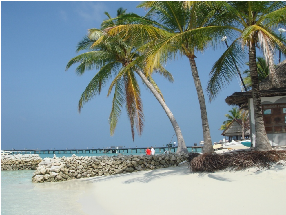
Plate 2: Two groynes which had been constructed using coral on western side of the island
