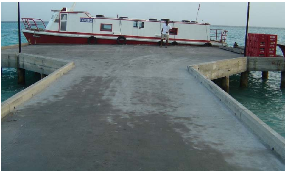
Figure 2: Existing Service Jetty looking towards the lagoon. The jetty head is of hexagonal shape to increase the length of the 'quay-wall'.
