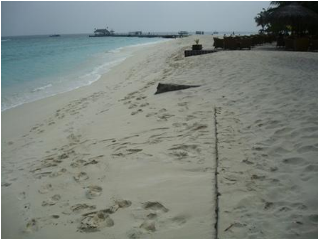
Figure 21 At present major accretion is observed at the eastern and south eastern side of the island, in the figure the it can be seen that accretion height has exceeded the height of existing retainment wall at this area (north of main jetty)
