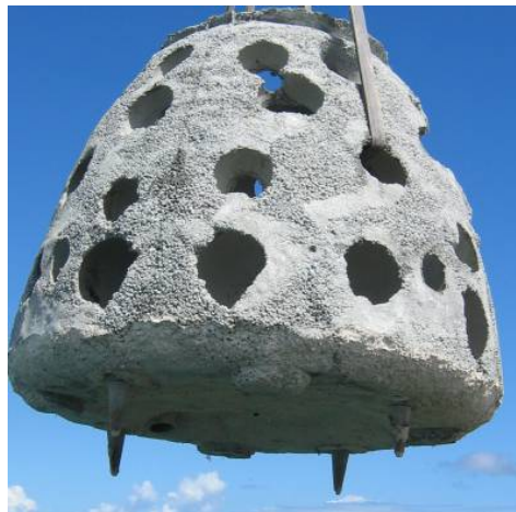
Figure 5: cross-section of a reef ball to make a breakwater
