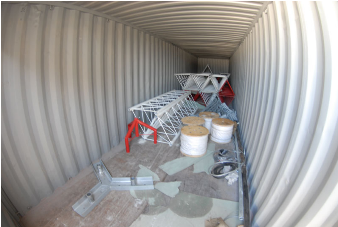
Figure 3: The met mast is delivered on site in sections in a container. Once the foundations are in place, they will be fixed on top
