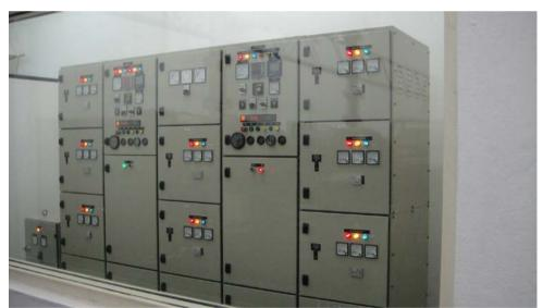
Figure 7 Panel board used at the powerhouse
