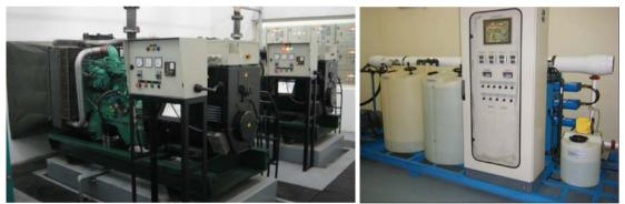
Figure 1 Generating sets and desalination facilities uesd at the island
