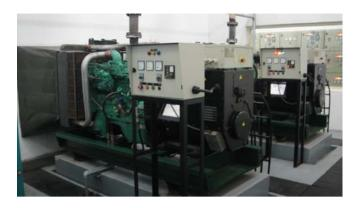
Figure 4 Diesel generating sets used at the island
