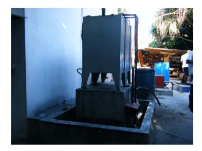
Figure 6 Day tanks located outside the powerhouse
