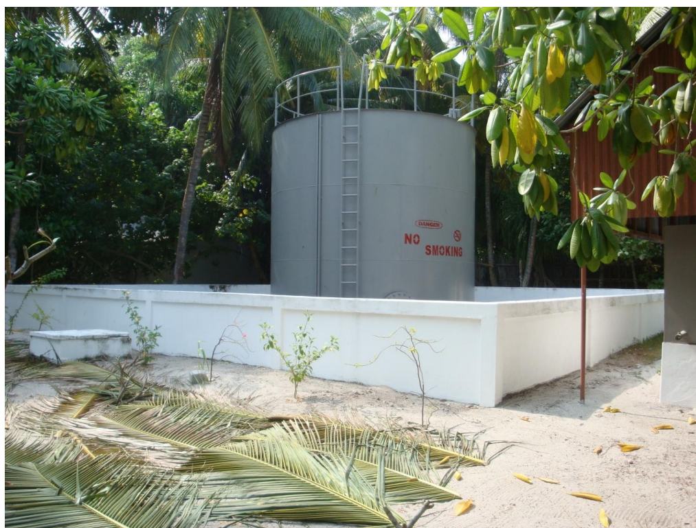
Figure 2.4: Fuel Storage Tank with bund
