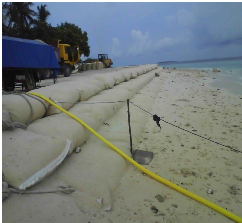
Figure 4: A beach protection revetment installed in R. Maduvvari using Elcorock containers
