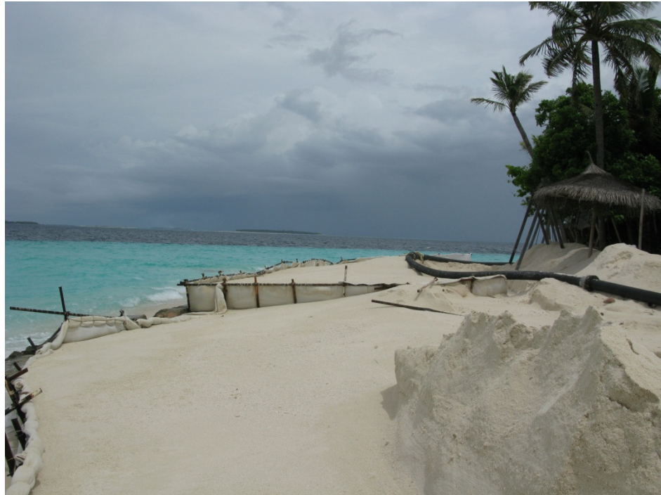
Figure 26: Geo-textile pockets retaining the sand on the south-western corner of the island
