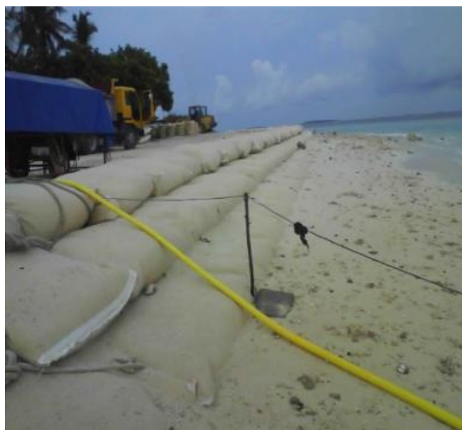
Figure 21: A beach protection revetment installed in R. Maduvvari using Elcorock containers
