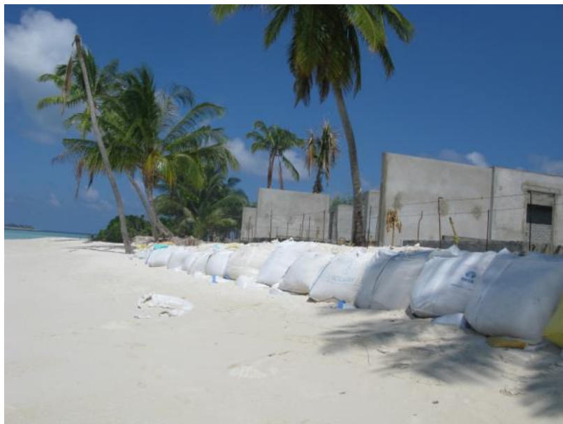
Figure 14: Sand bags deployed to retain the beach. The picture was taken during low tide.
