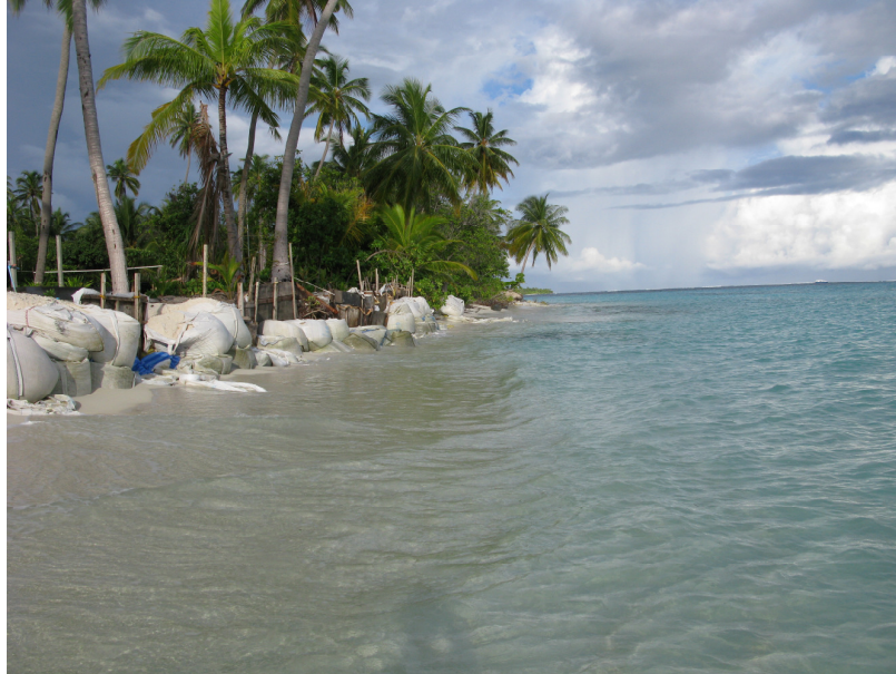
Figure 5: Ad hoc solutions to counter erosion on Magudhdhuvaa
