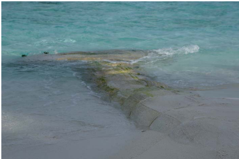
Figure 4 Sand Bag Groyne constructed in the island
