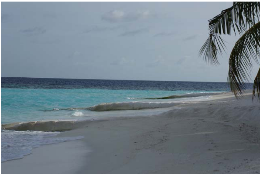
Figure 7 Groyne Field along the shoreline
