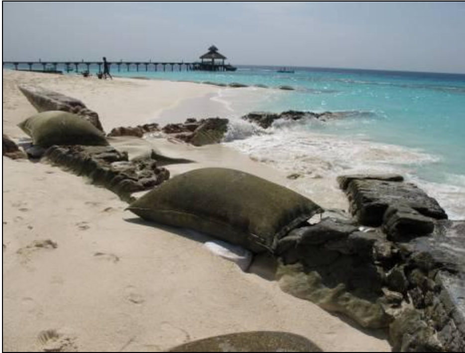
Figure 2: Existing coastal erosion protection at Reethi Beach Resort.
