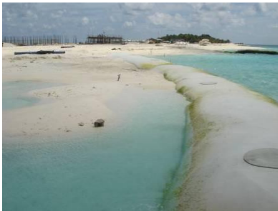
Figure 5: A beach protection revetment installed in K. Bolifushi.
