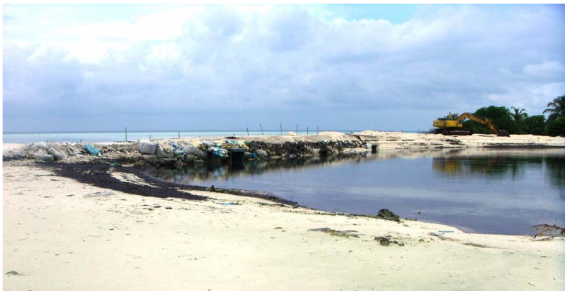
Figure 1 Existing causeway constructed by the contractor for the resort development project
