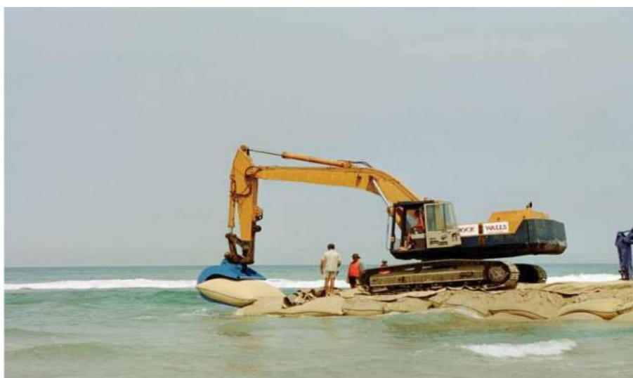
Figure 29: Placement of geobag using excavator (Source: Elcorock)
