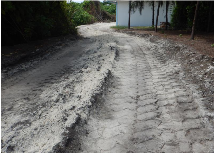
Figure 24: Impact on roads from heavy vehicle transport in an island in Maldives
