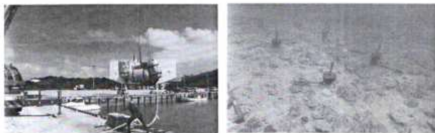
Figure 4: Unloading of the WEC units and metal rim and shafts attached to the holes drilled for WEC mounting
